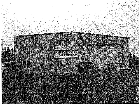
Bemidji, Minnesota Facility North Central
