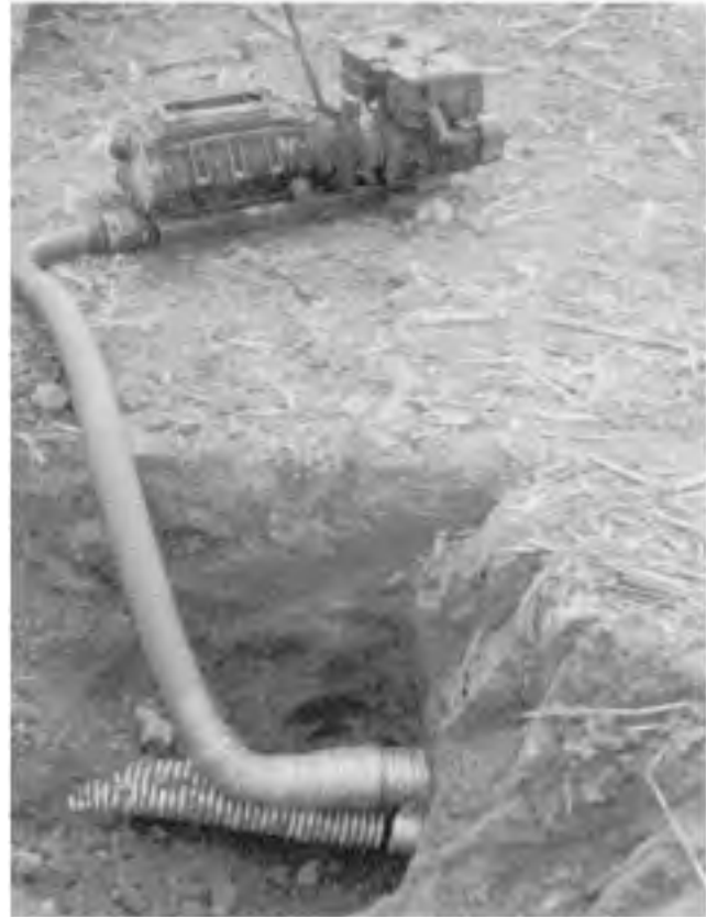
Fig. 1. Turbine blower used to force smoke into the tile line.
